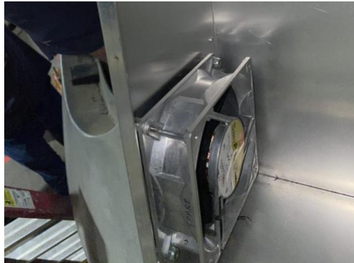
Figure 76: Spare Fan inside Electrical Box
