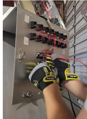
Figure 51: Checked Wire Continuity
